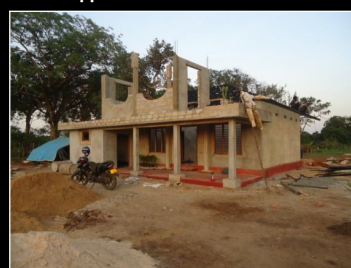
NHDA Building - Mullaitivu
