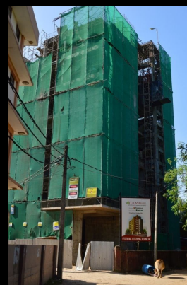
Construction of Condominium Housing in Jaffna
