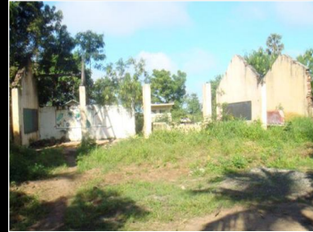
Parappukandal School in Mannar
