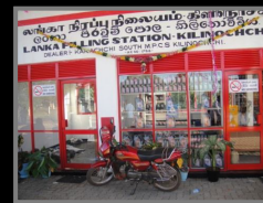
Re-Establishing Filling Station - Kilinochchi
