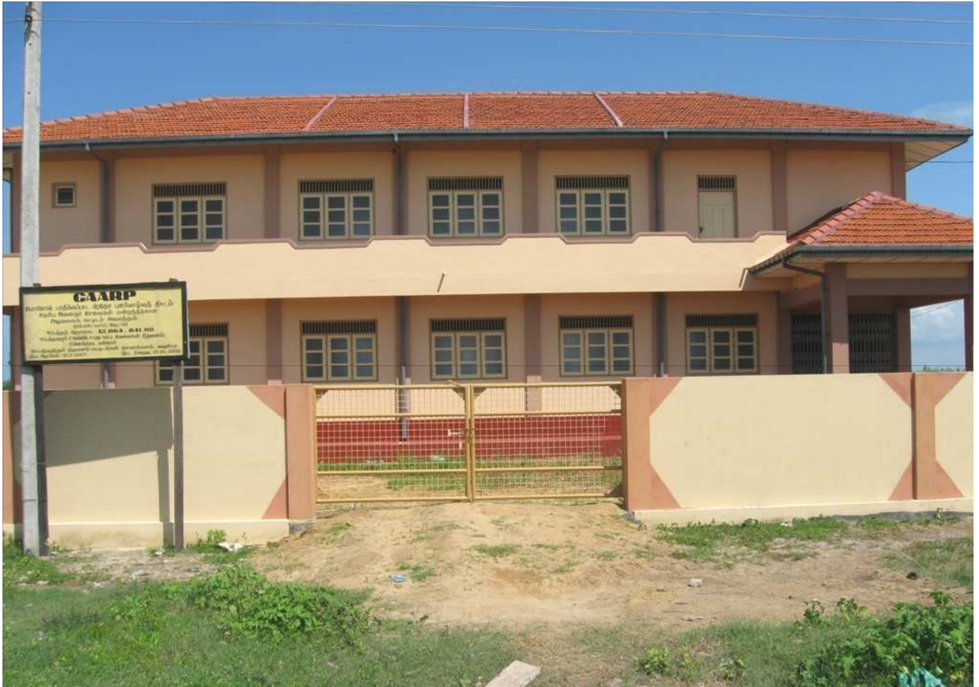
OFFICE BUILDING, NATIONAL YOUTH SERVICE COUNCIL, MANNAR
