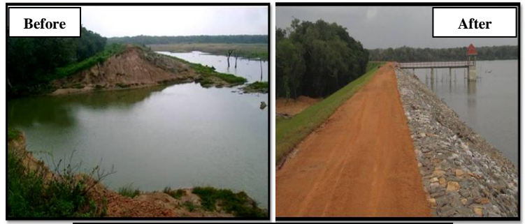
Restoration of Kalmadu Tank - Kilinochchi
